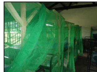
Mosquito nets installed at Makobore high school
