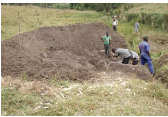
Digging the reservoir
